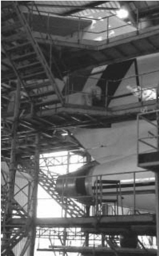
Photograph A Engineer working on staging
